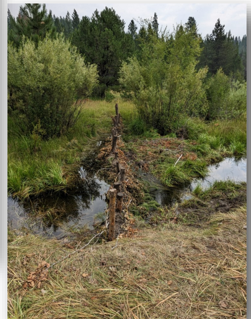
Picture 4: Fully constructed BDA from picture 2.
