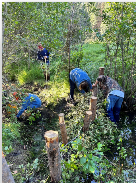
Picture 3: Youth crews construct BDA by weaving materials through posts.
