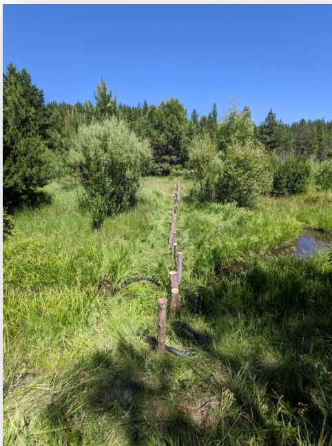
Picture 2: Posts installed across channel for future BDA.
